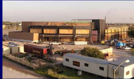
Construction Progress October 2004
