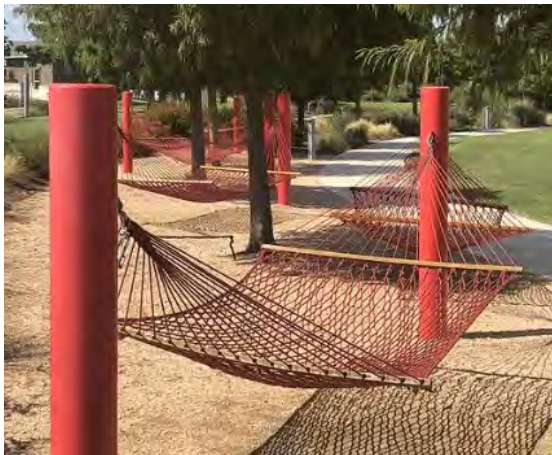
Hammock Posts at Courtyards Custom Steel HSS Round post, powder coated black or purple Height: 54" to 60"
